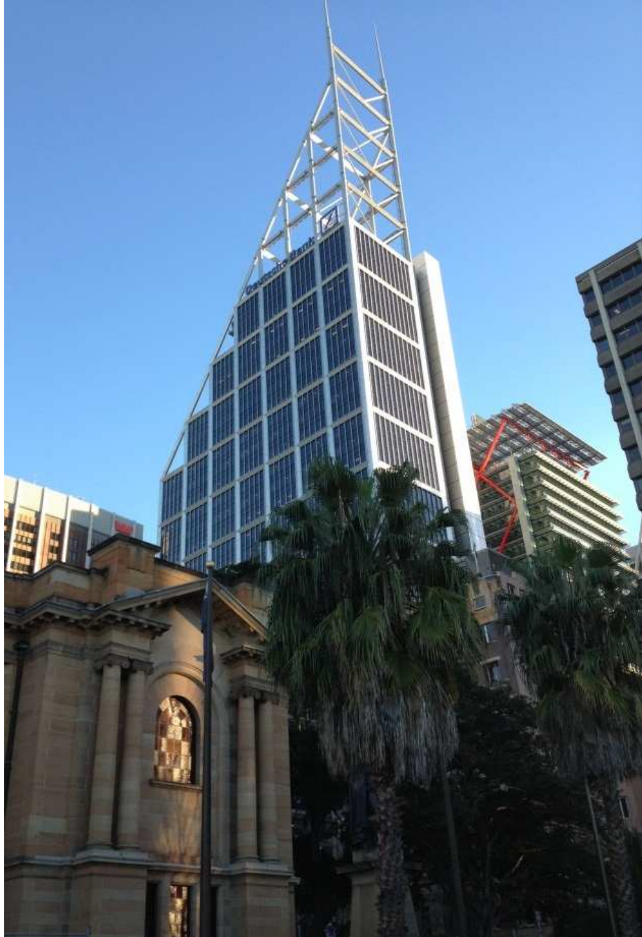
Figure 15 – 126 Phillip Street Source: JBA
